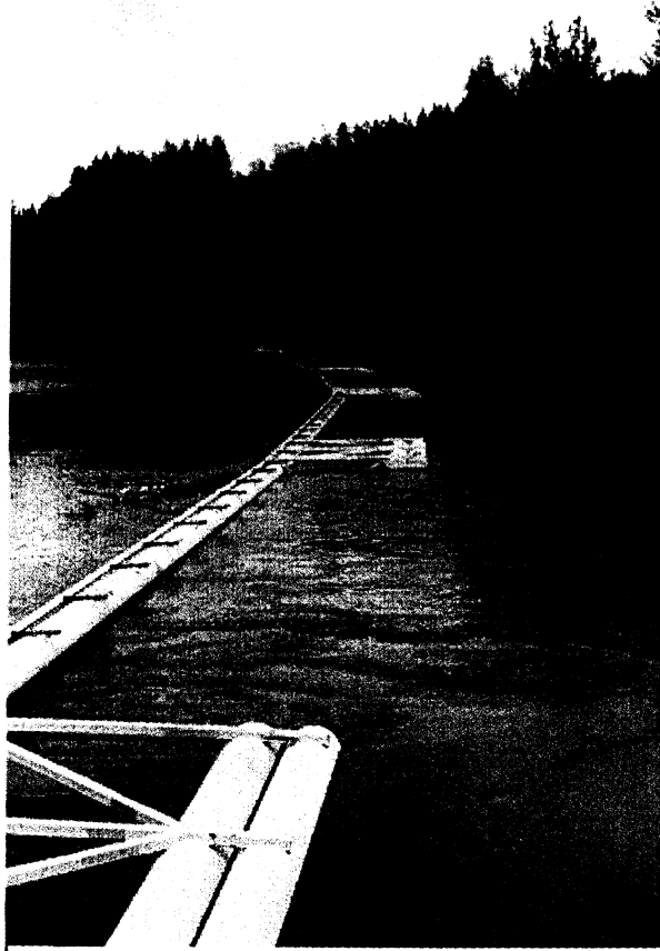
Figure 2. Ice boom at the Keltti hydropower station. Earlier the boom was used for log floating in River Kemijoki.
