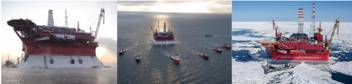
Figure 2. Concrete GBS: Prirazlomnaya, Pechora Sea, Russia (courtesy of GazProm)
