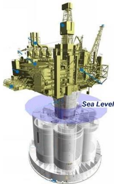
Figure 6. Hebron platform concept, Jeanne d’Arc Basin, Canada (from Widianto et al., 2013)
