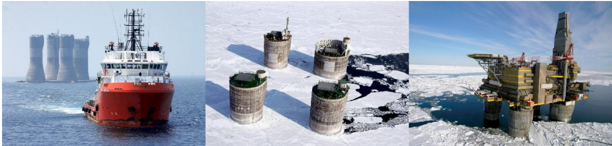
Figure 3. Concrete multi-legged GBS: Lunskoya-A, Sakhalin (courtesy of GazProm)
